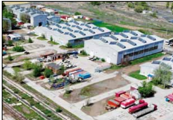
IGS' High Tech fabrication facilities, shops and warehouses with 3 railway connections. IGS' base is in close proximity to Karachaganak Oil & Gas condensate field.
